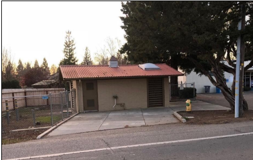
Figure 5 - Durham Irrigation District – Well #4
