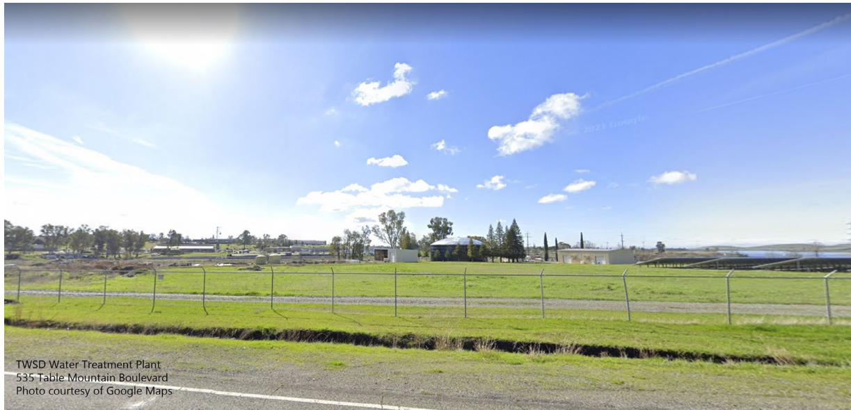
Figure 7-11: Water Treatment Plant - Existing Site
