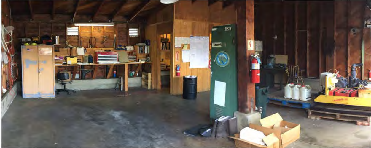
EXISTING OROVILLE MOSQUITO ABATEMENT DISTRICT BUILDING
