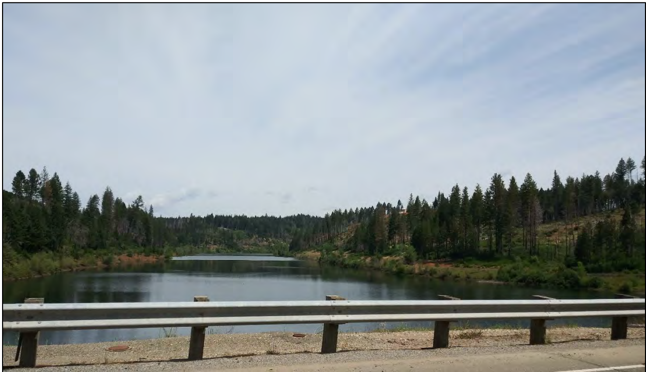
Figure 7.14: View of Magalia Reservoir
