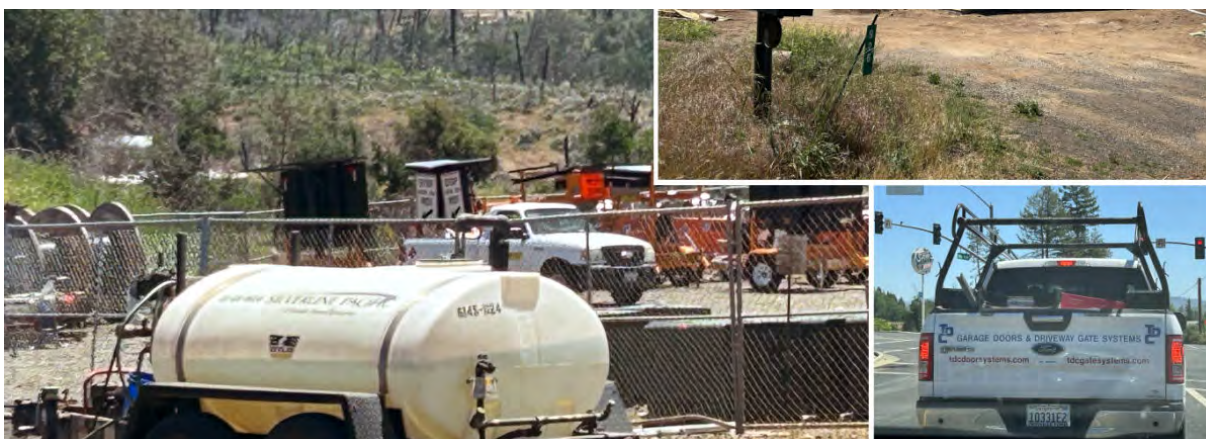
Construction work was widespread in mid-May 2023. Felicity Barringer
