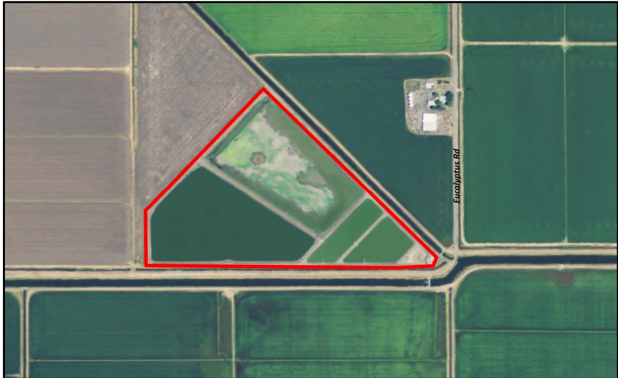
Figure 3-2 Richvale Sanitary District Wastewater Treatment Facility Aerial Photograph
